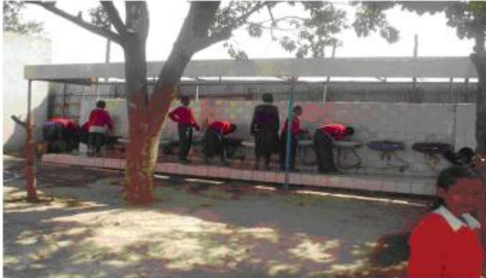
Figure 6.2 Drinking taps and hand washing basin arrangements in a school.
